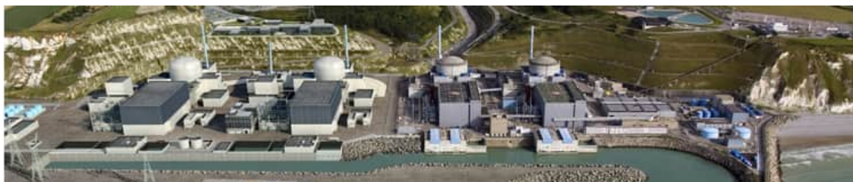
Site EDF de Penly.
